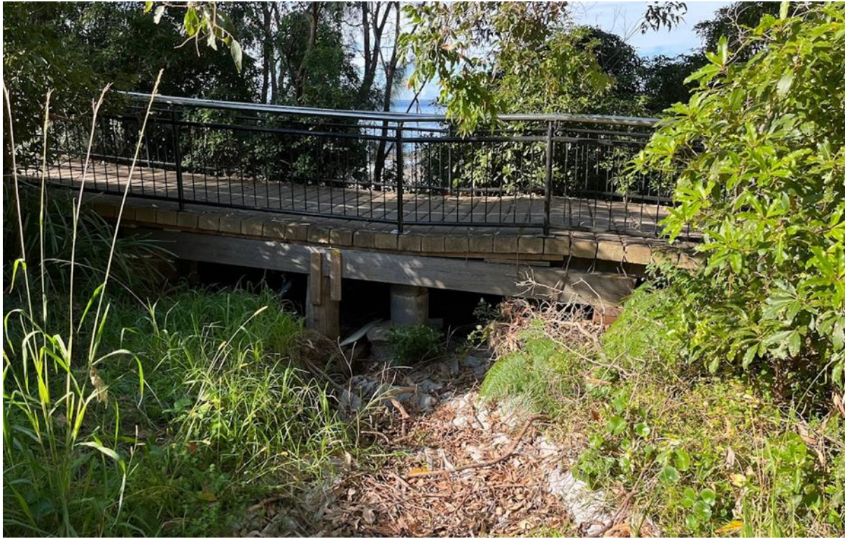
Photo 5: Surface underneath the boardwalk where the existing geofabric would be removed and replaced with jute mesh and rock rip rap armour.
